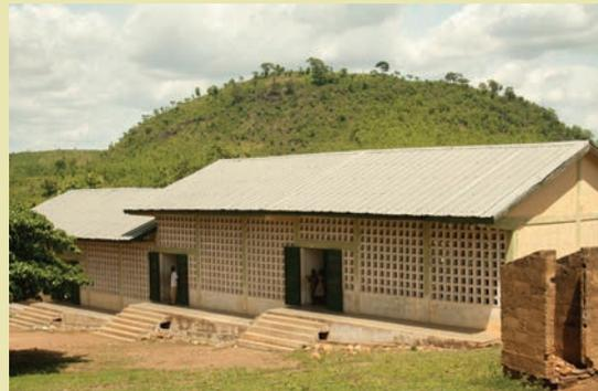
Traditional *apatam* classrooms (above left) are constructed from grass and leaves. The new ones (above right) have high roofs to keep them cool, while hollow lattice walls provide light and ventilation.
